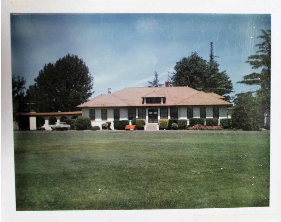
Figure 19: Women's Building with colonnade left of frame, 1973, on file at Napa County Building Department.
